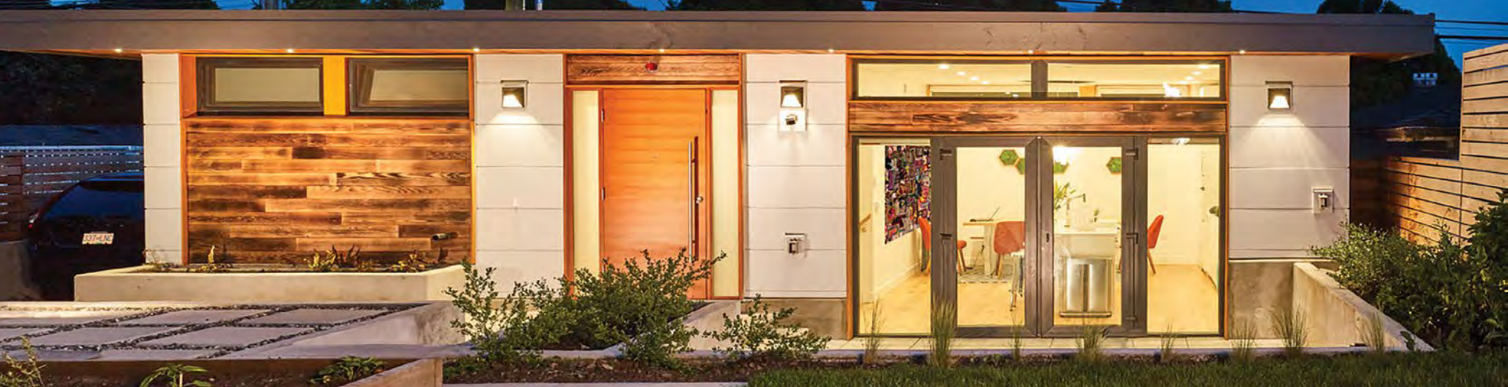
Photo: Lanefab Design/Build
